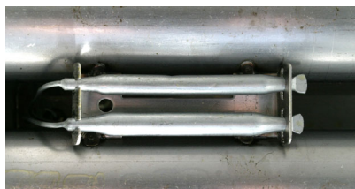
Typical high-limit/sensor probe locations and mounting hardware.
